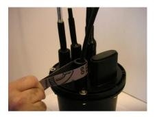
Warming of cable-entries till they get black. Starting from lower shrink the tube shortly, wait approx. 1-2 minutes, till the tube holds on the entry, and continue from top to closure lid.
