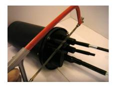
Napping of cable- and entry surface with attached Abrasive. Fix Kevlar and reinforce-element on the Strain relief bar.
